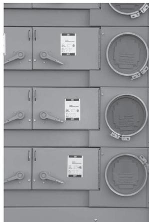
**FSMC Units Installed in Pow-R-Line C Switchboard**
